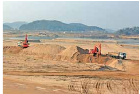
Plate 2. Dredging work for the FMRRP already in full swing, February 2010.
